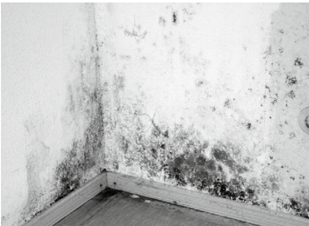
Fig. 5: Example of mould infestation in a corner
