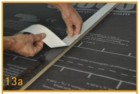
Apply TESCON® NAIDECK and Position Battens Remove backing paper from TESCON® NAIDECK and place the counter batten in position to align with the rafters or trusses underneath.
