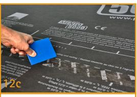
Apply TESCON EXTORA® Using the PRESSFIX Tool
