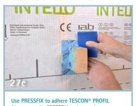
Always use the PRESSFIX tool to apply pressure to the adhesive to ensure durable adhesion.
